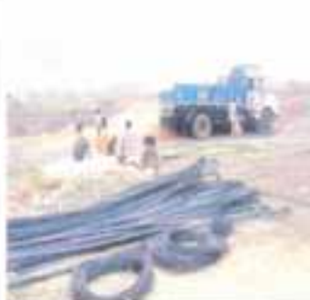
Bringing in building material
